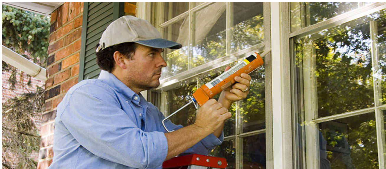
Window Caulking, Source: osceolagenerations.org
