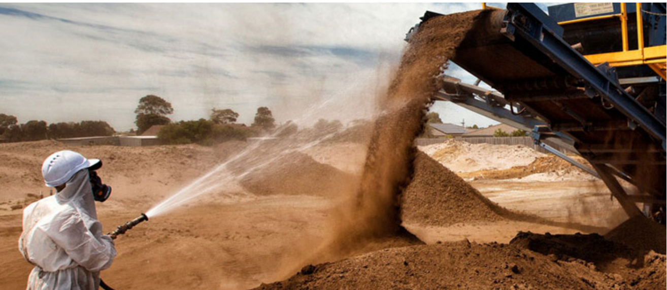
Treating polluted soil using bio-remediation technique, Source: AL-DHOW
